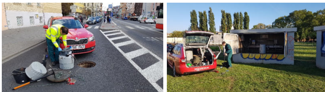
Fig. 29: Installation and operation of automated ISCO samplers
