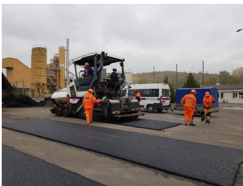
Fig. 16: Photo of the laying of test surfaces made from the developed materials
