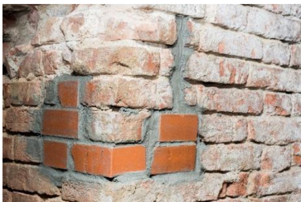
Fig. 5 Walled-up opening
