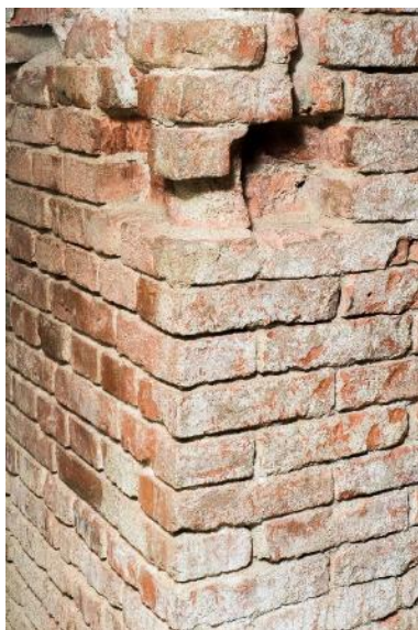
Fig. 1 Masonry prepared for the application of remediation materials
