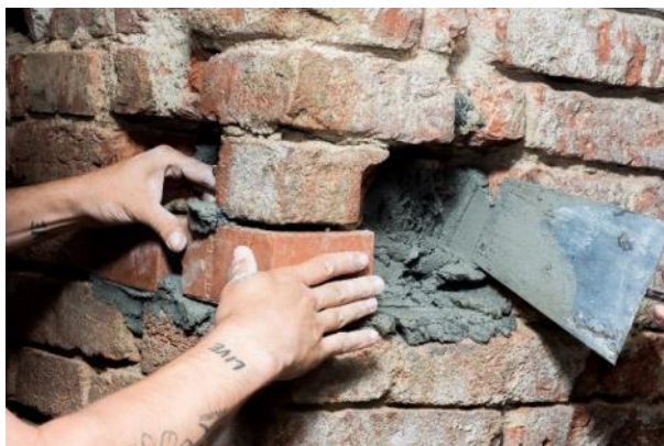
Fig. 3 Laying of the bottom row
