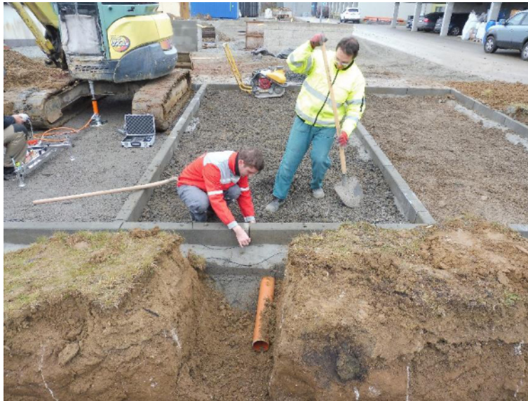
Performance of static load tests (left); installation of moisture sensors and a drainage system (foreground)
