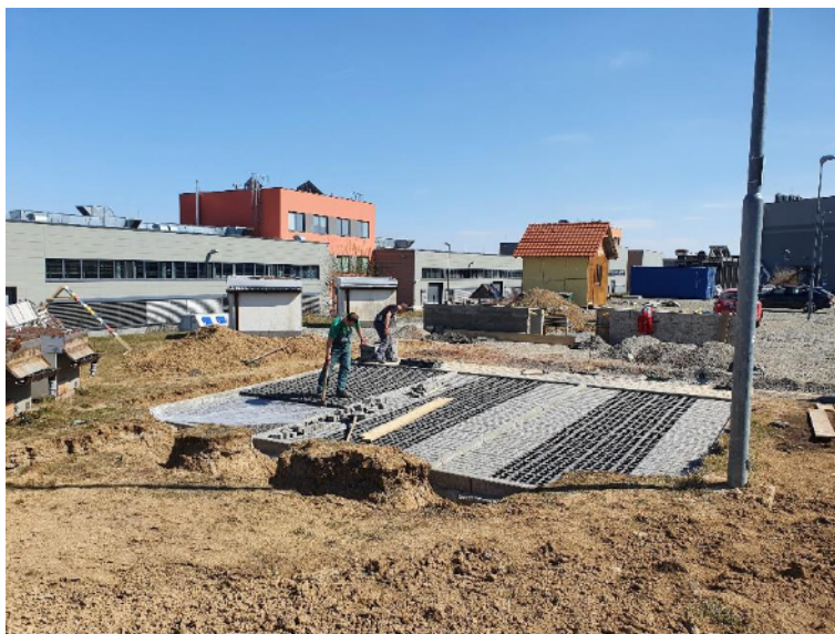
Filling in the grid with concrete blocks; preparation for the planting of a lawn
