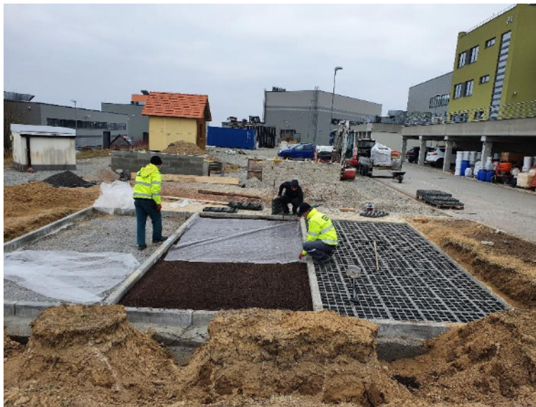
Installation of AS – TTE soakaway grids
