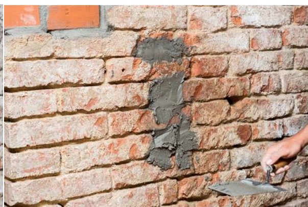
Fig. 6 Application of repair mortar
