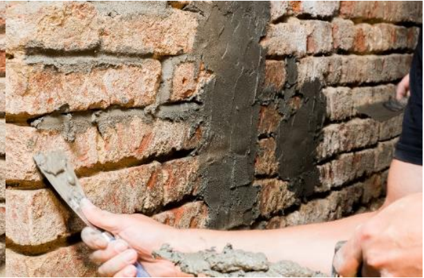
Fig. 8 Masonry grouting
