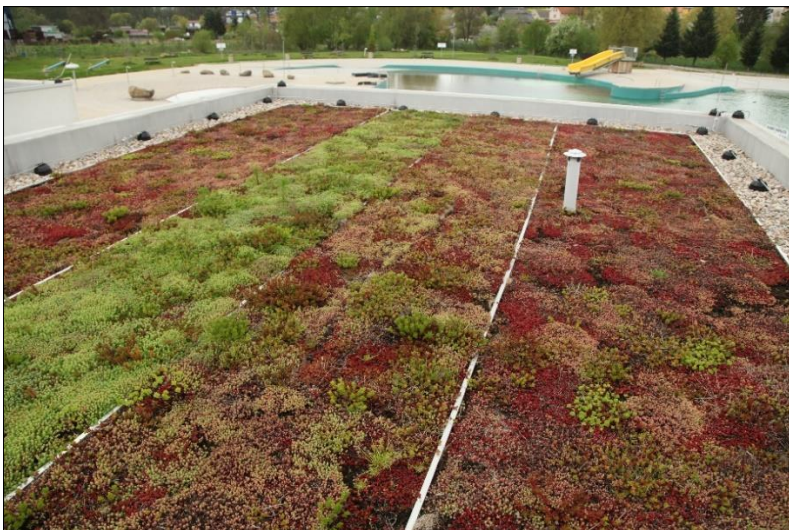
Figure 4. Experimental green roof amended with biochar
